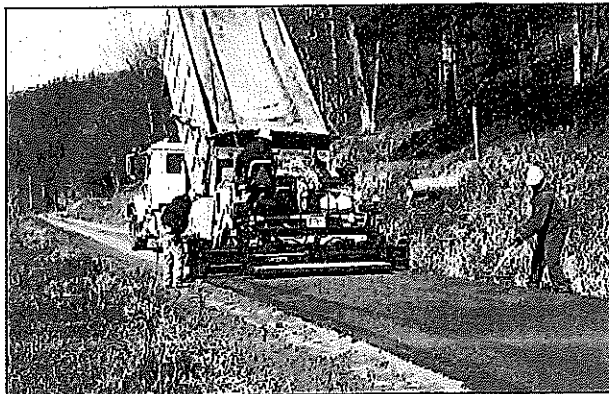
Paver-placement of TSA is preferred for longer sections of trail as pictured above.
